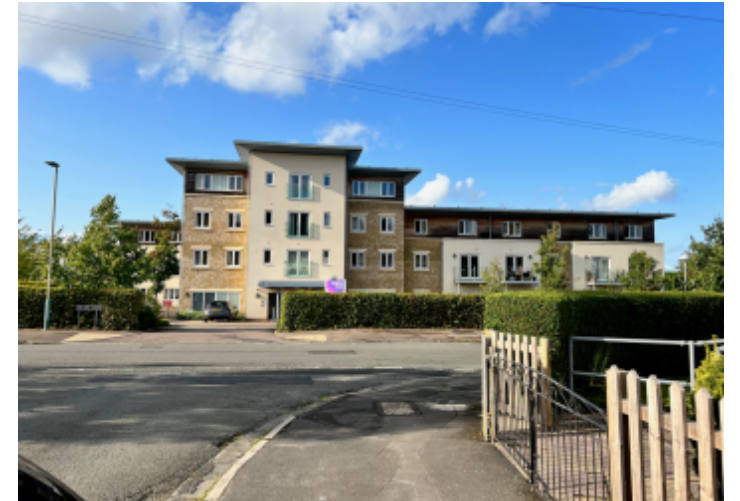
Middleton House care home in Pilley Lane to east
